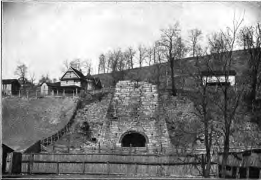
FIG. 1.—RUIN OF BLAST FURNACE, LONACONING, ALLEGANY COUNTY.
